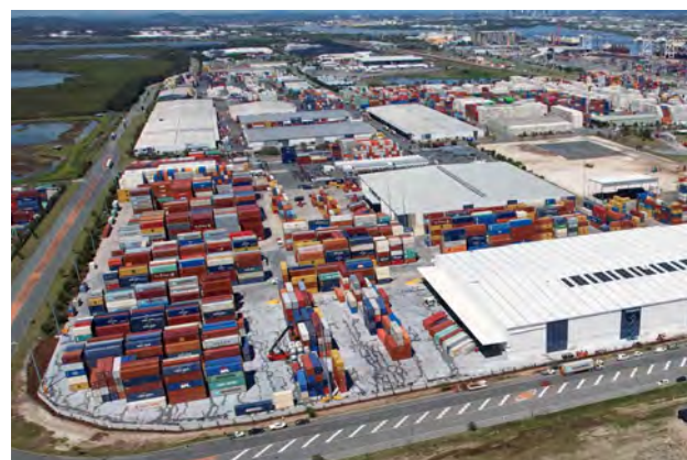
AEI works completed in 4Q2022
