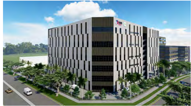
AEI works expected to complete by 1Q2024
